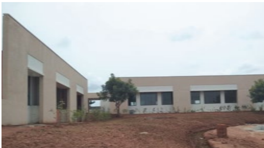
A partial view of the Laboratory Block at the Shivanapura Campus
